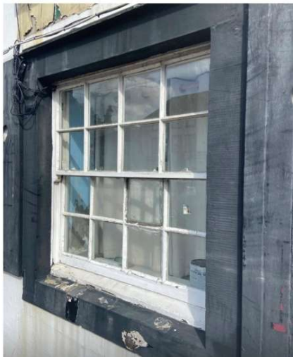
Picture 1: ground floor window, current condition
