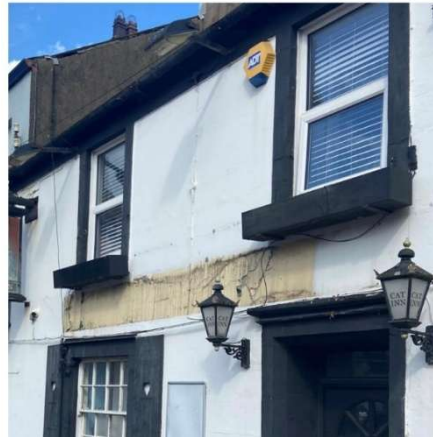
Picture 2: Frontage, ground floor and first floor. First floor UPVC windows previously installed, before I became owner.
