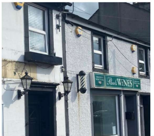
Picture 3: Showing Adjacent building with upvc windows.
